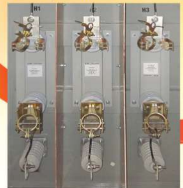
Factory mounted arresters
