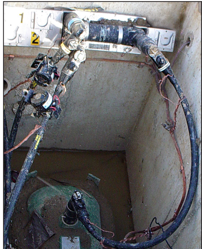
▲ Typical installation showing a 3-position feedthrough application in a submersible vault.
