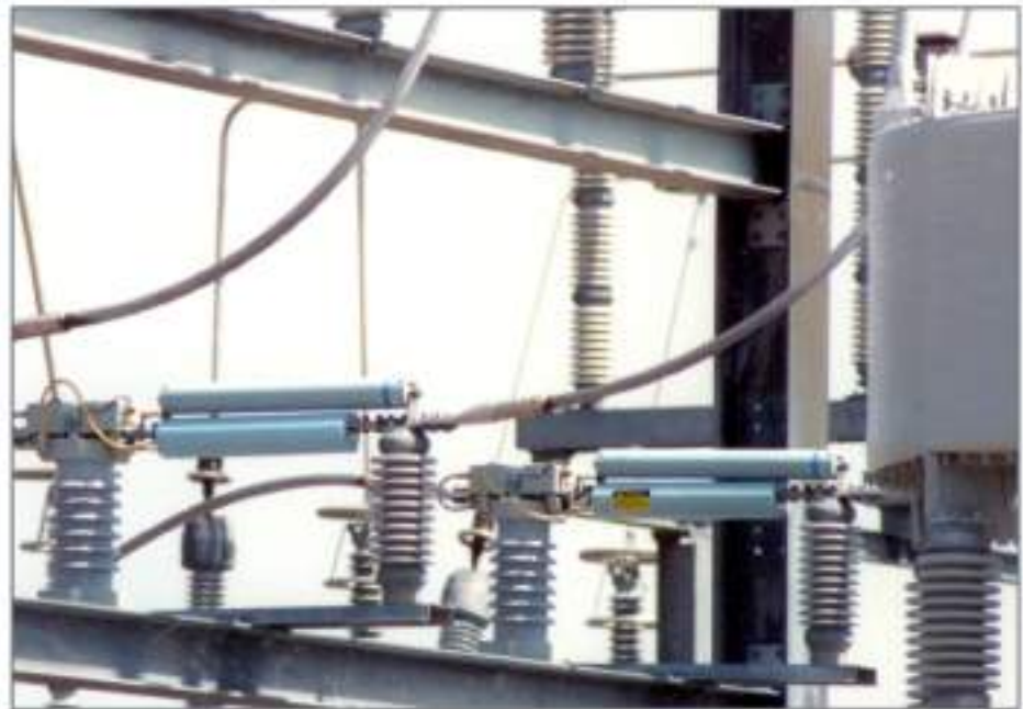
▲ Structure mounted 38kv, 1200A CLiPs in a reactor bypass application.
