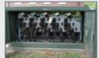
SF6 Underground Distribution Switchgear
