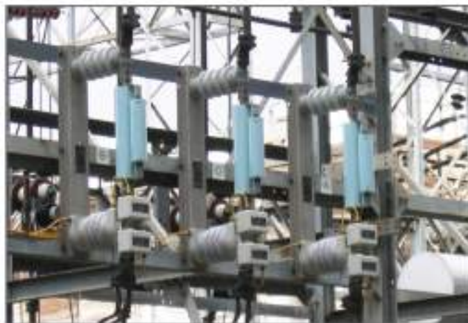
◀ A substation CLiP protecting a government facility.
