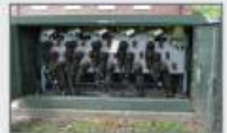
SF6 Underground Distribution Switchgear
