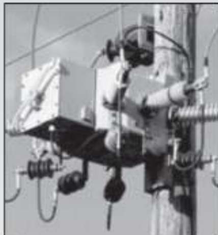
▲ RP style switch with motor actuator.
