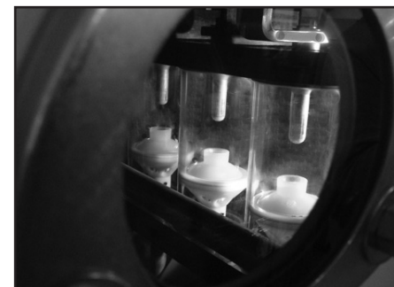
▲ Load break switch visible break.
