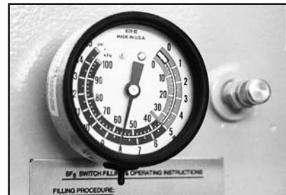
▲ Pressure gauge and fill valve
