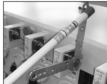
▲ Interrupter with hotstick operable handle.
