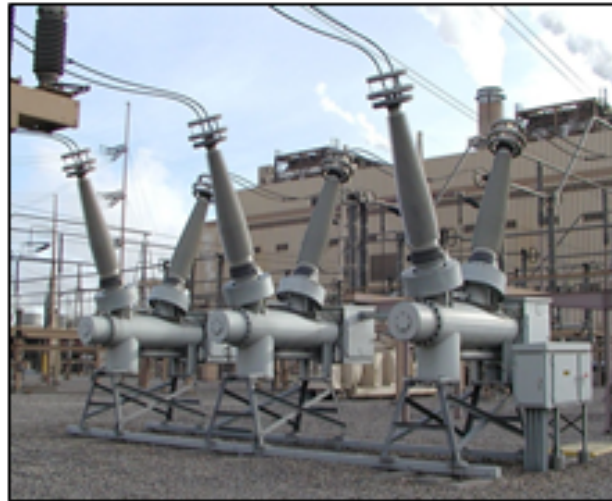
HHI-R 362 kV/50 kA with PIR
