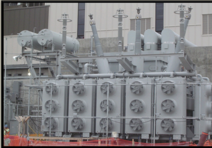
MidAmerican Council Bluffs Energy Center Unit 4 24/345kV 1,036MVA GSU Year of 2005
