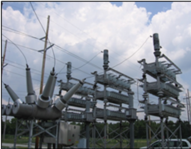
HS-R 145 kV/40 kA with PIR
