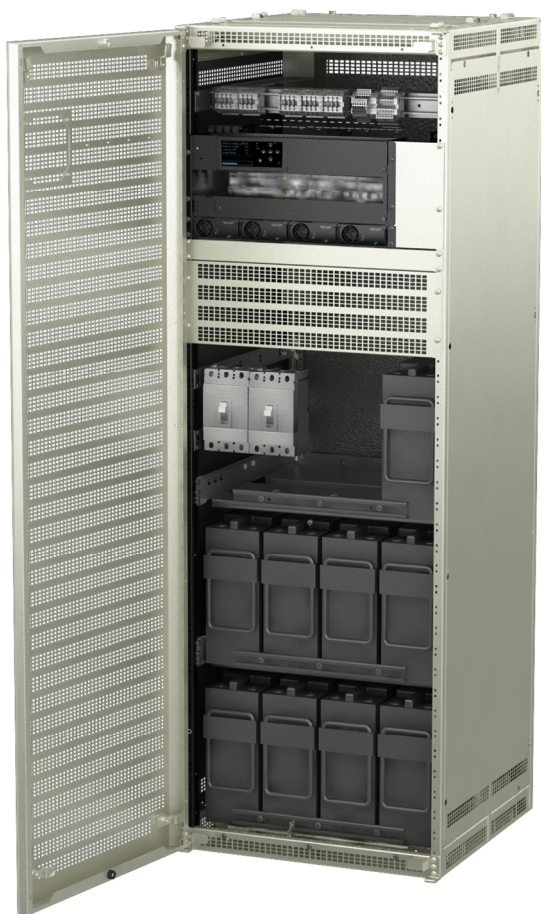
IBB SYSTEM IN FPC CABINET
